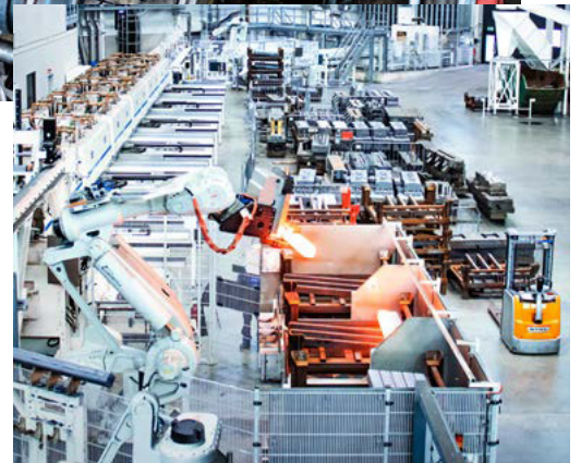
New plant concept of induction furnace supplemented by holding furnaces helps boost energy efficiency.
